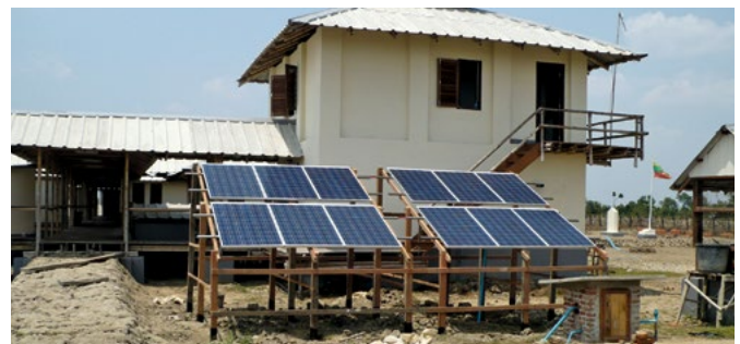
Power supply to a hospital
